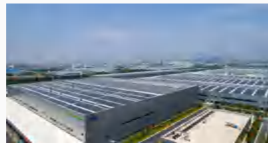
Hefei GCL SI Xinyu PV Power Station
